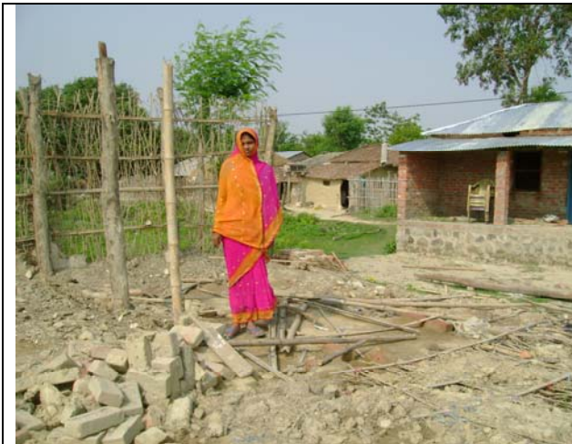
Facilitator Rekha Kumari Mahato standing on the ground where the center was built. The building collapsed by wind during the session and the classes were run for a while in the club house which is seen at the corner.
