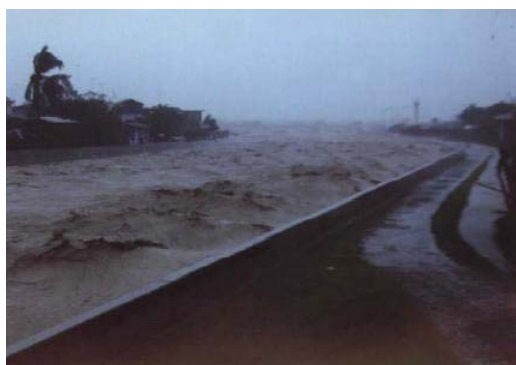
Concrete-type revetment in Ormoc City
