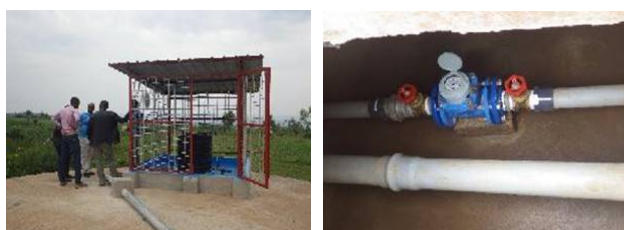
Photo 3 The disinfection facility installed by the pilot construction (left), a water meter (right)
