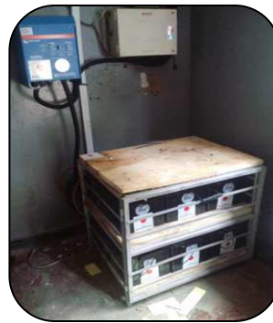
Inverter, Battery Box, and 6 Batteries
