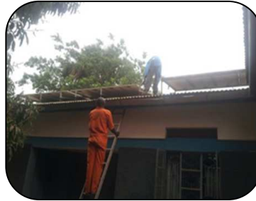
Installing 8 solar panels at Kitgum DWO
