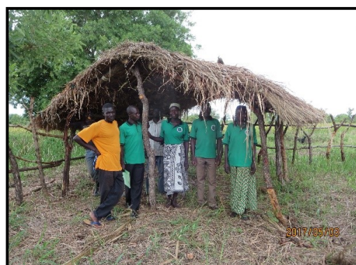
Construction of Kraal and Shed (Atiak S/C)
