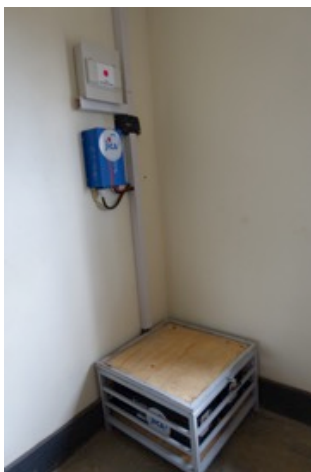
(Left) An Inverter and solar batteries in a battery rack in Dranya S/C
