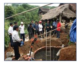
Visitors also learned how to build the biogas system, including making hole, building main pressing digesters. installing digesters, pipeline systems, safety valves, using biogas kitchen and light.
