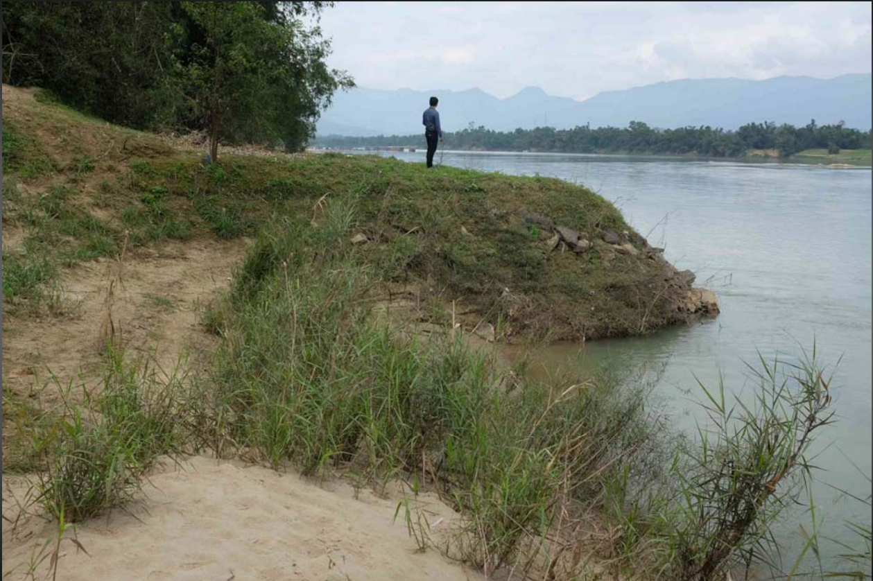
Masonry groyne 4 years after construction
