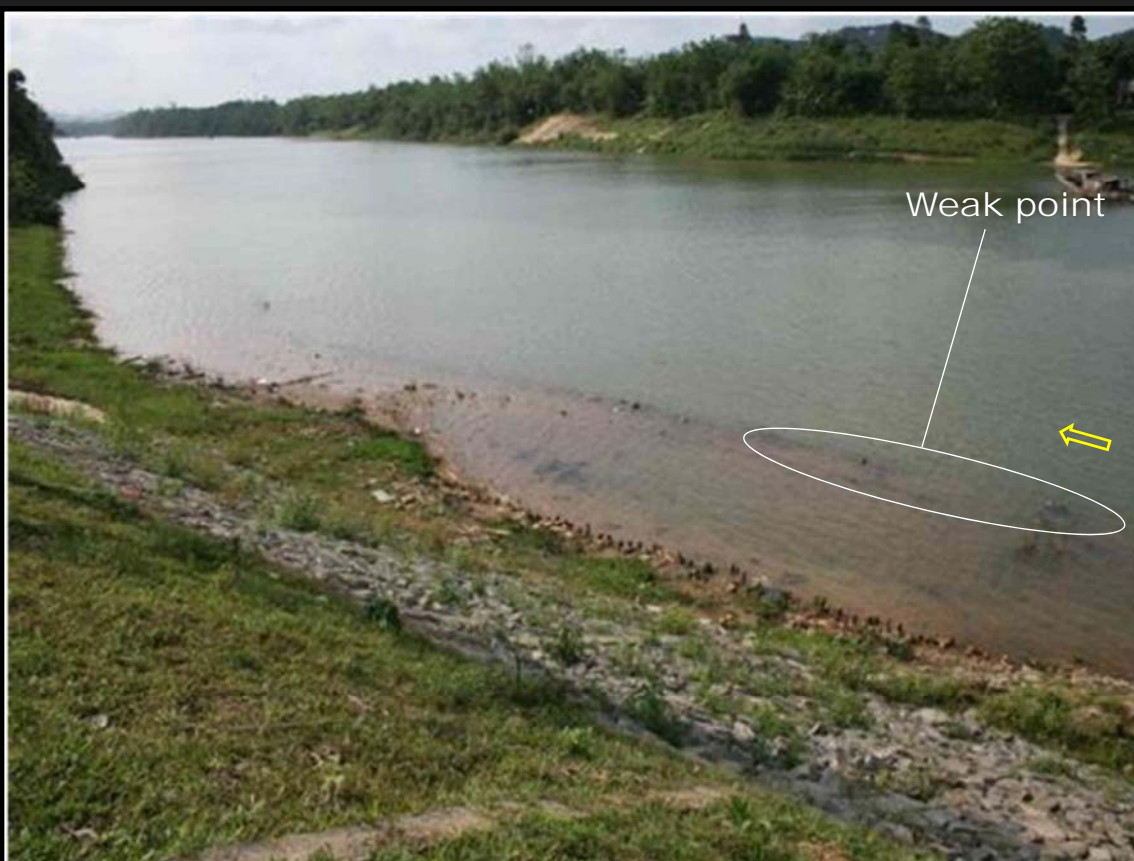
Bamboo dragon mattress 2 years after construction (2012)
