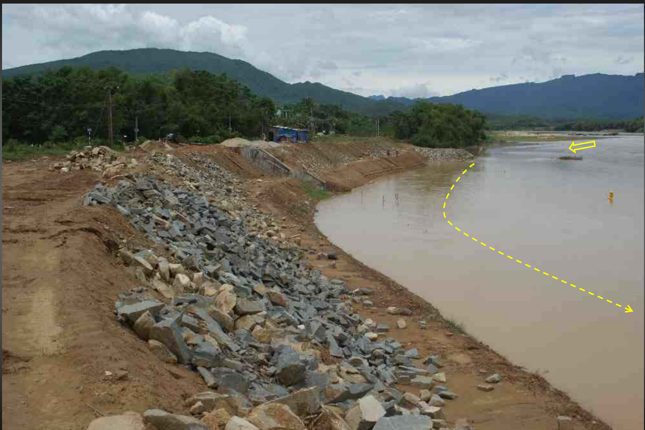
Bamboo guide wall under the water (Thanh Xuyen, 2010) (2010)
