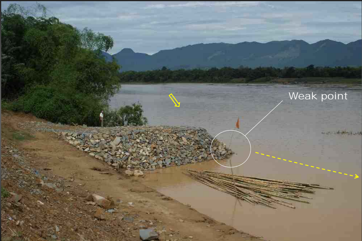
Masonry groyne completed (Thanh Xuyen, 2010)
