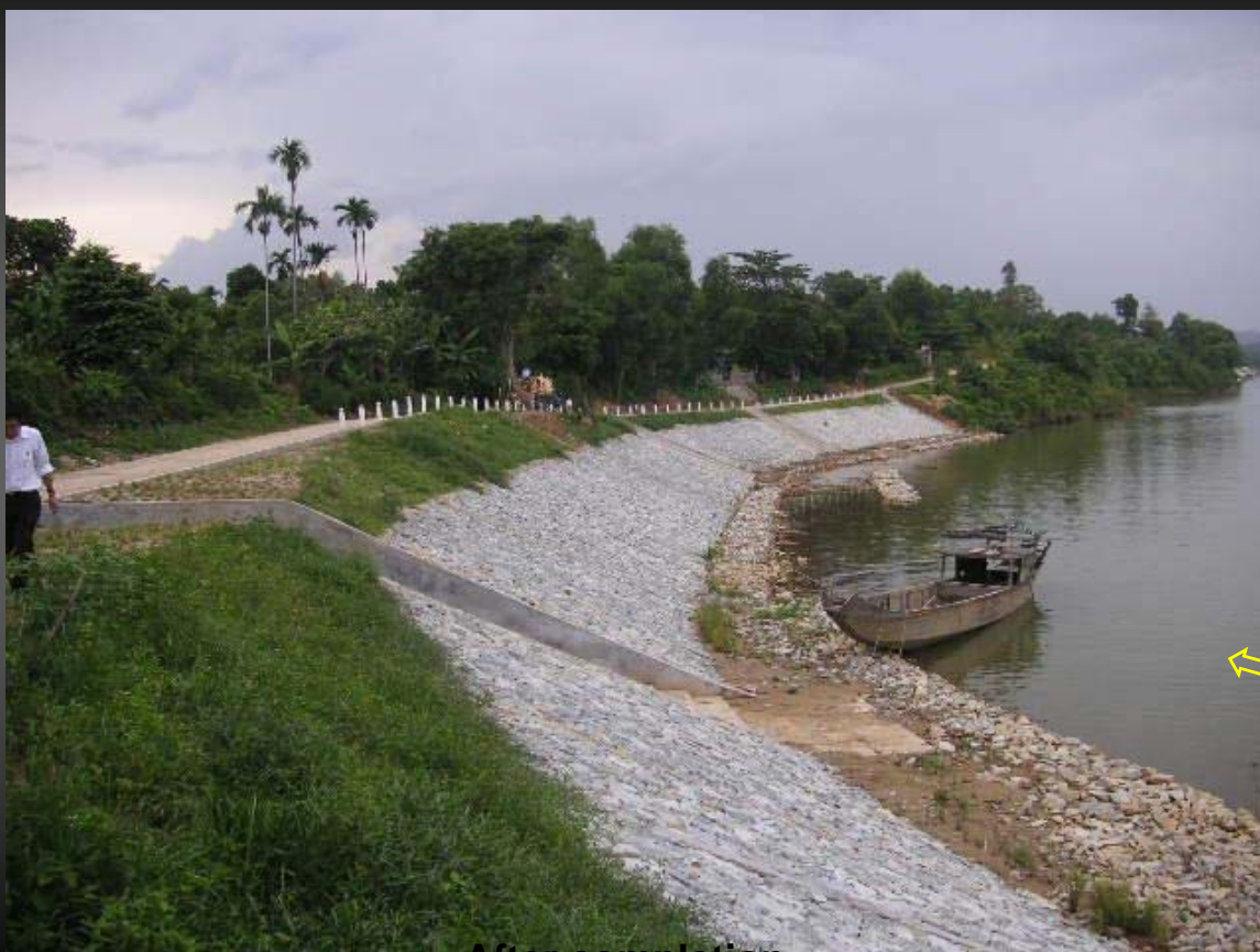
Rebetment completed with bamboo dragon (2010)
