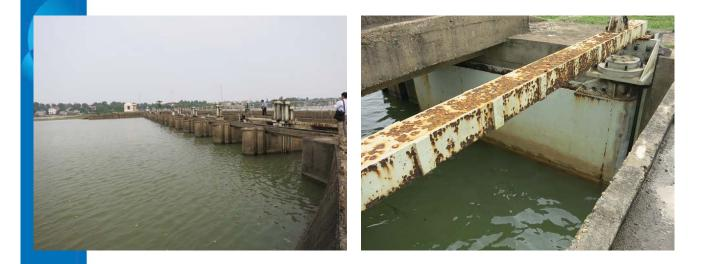
Tidal weir, especially metal gate become old for work. Rehabilitation and daily maintenace are needed.
