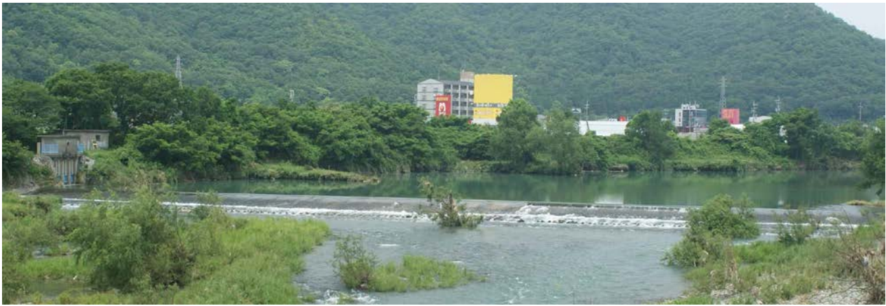
Groynes, Intake and Shikama Weir
