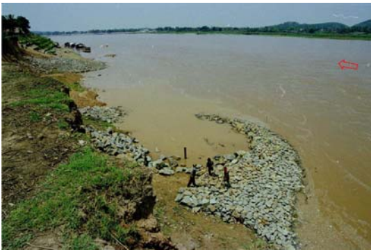
Photo 5 No.1 and 2 masonry under construction (May 1998)
