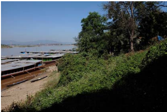
Photo 9 No. 1 groyne concealed by vegetation (February 2014)
