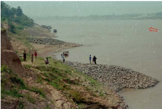
Photo 6 No.1, 2, 3 and 4 masonry completed (April 2000)
