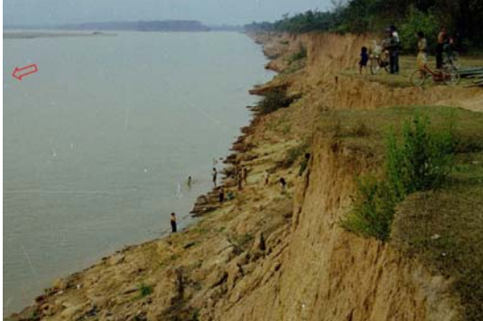
Photo 1 3km-long riverbank erosion (February 1998)
