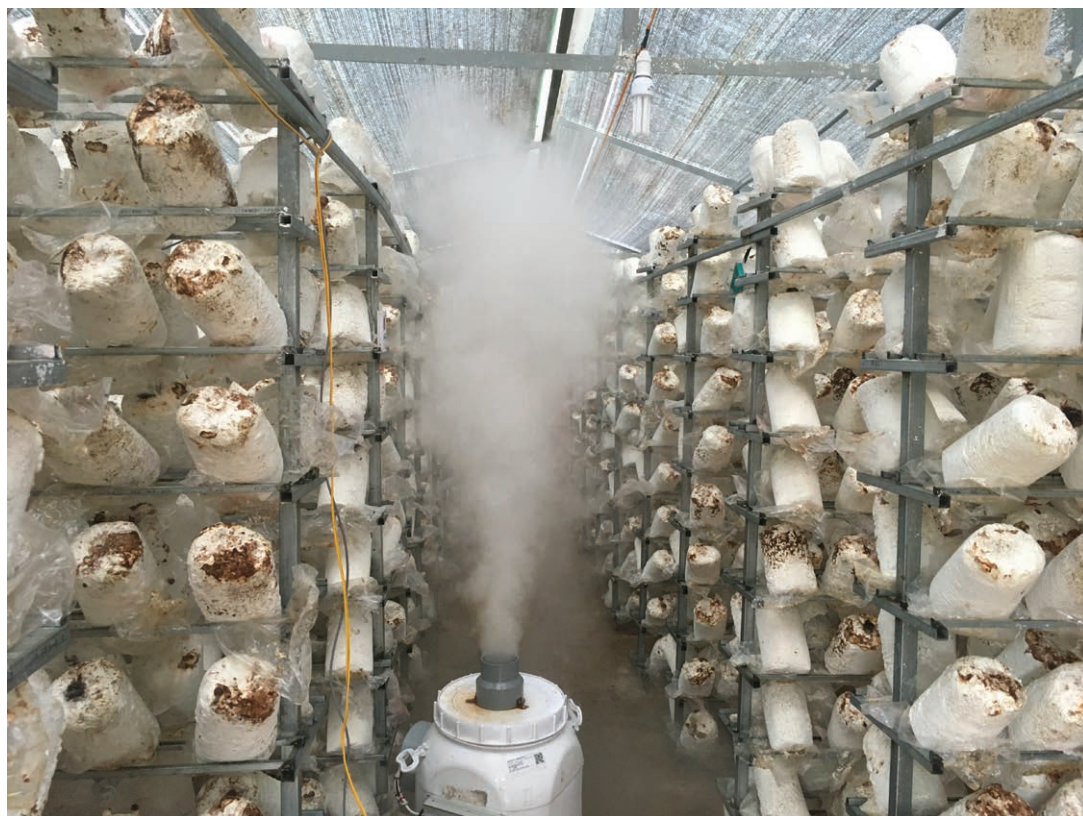
Installation of humidifier in the mushroom house
