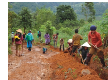
Villagers contributed labor for construction
