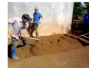
Working in construction of kids friendly toilet
