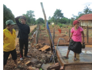
One water intake point was broken inside the hamlet,
