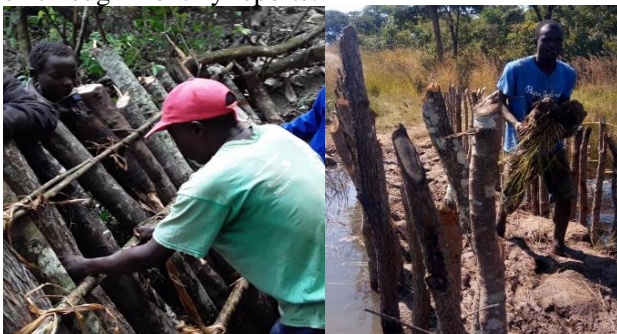
Inclined weir at Funda site (left: Mkushi district, Central province, 2019) Double line weir at Kazhimbe site (right: Mufumbwe district, Northwestern province, 2019)
