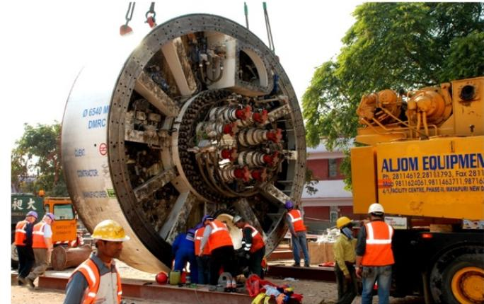
Assembling of a tunnel boring machine in Delhi Mass Rapid Transport System Project
