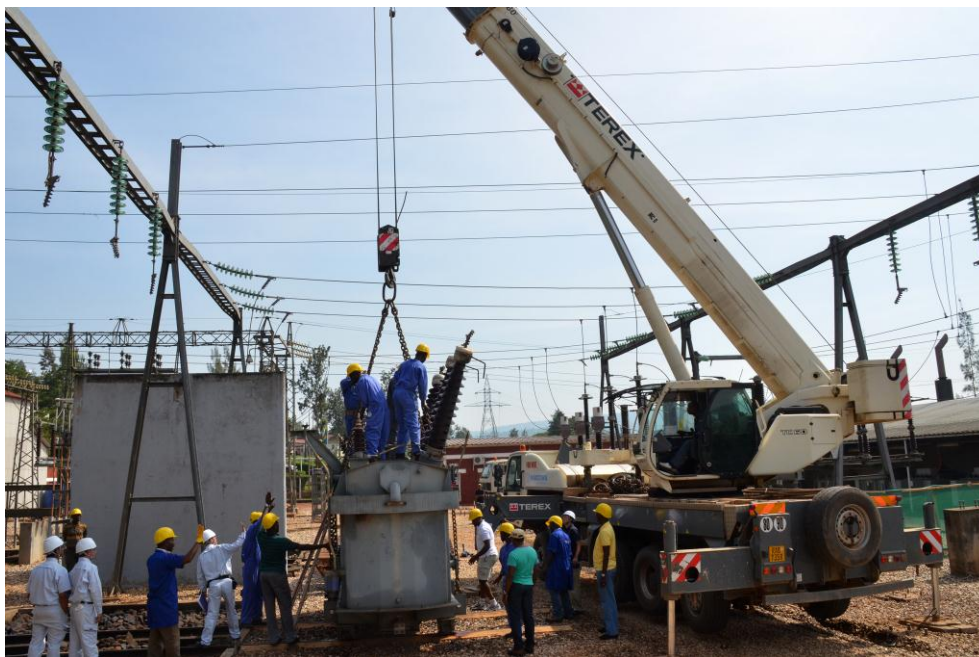
Jabana substation installation work
