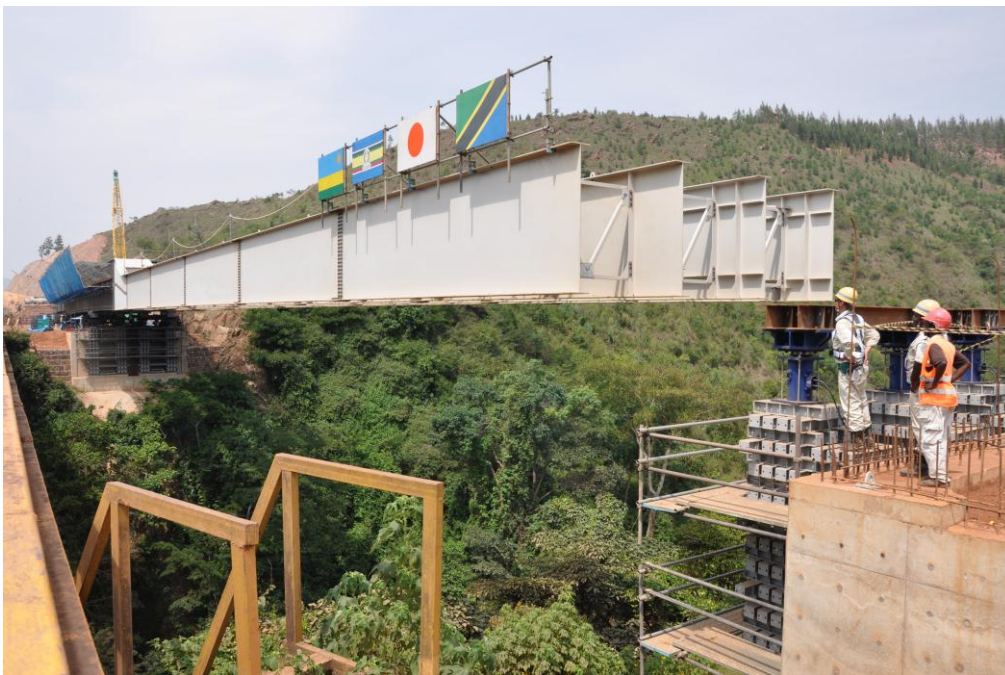
Rusumo temporarily bridge reaching Tanzania side
