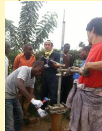
JICA W-SAT volunteers demonstrate how they repair hand pump
