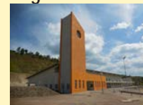
New building of OSBP facilities at Rusumo Border
