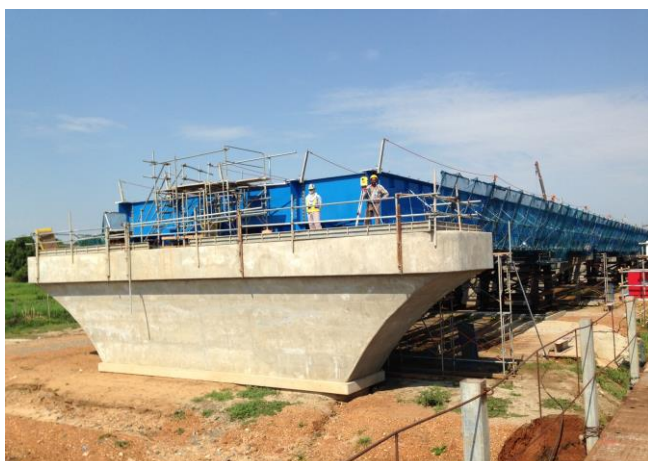
Construction of pier
