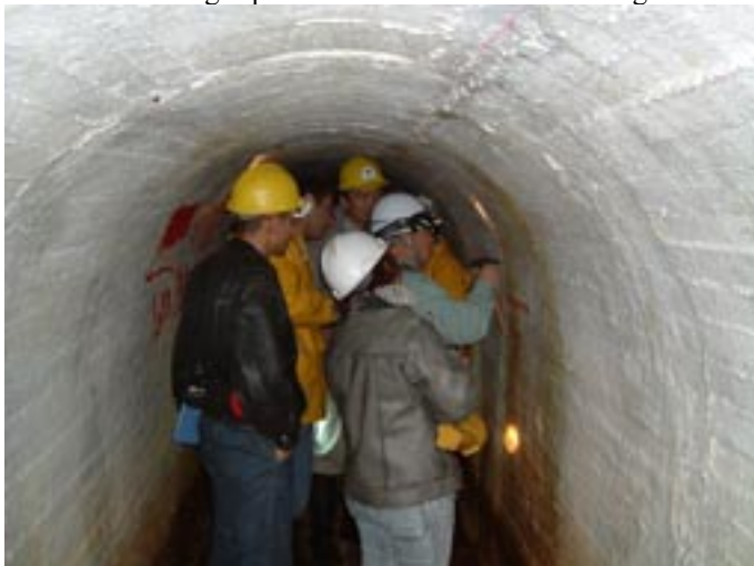
Japanese Consultant, Contractor, and DAWSSA staff discuss repairing techniques
