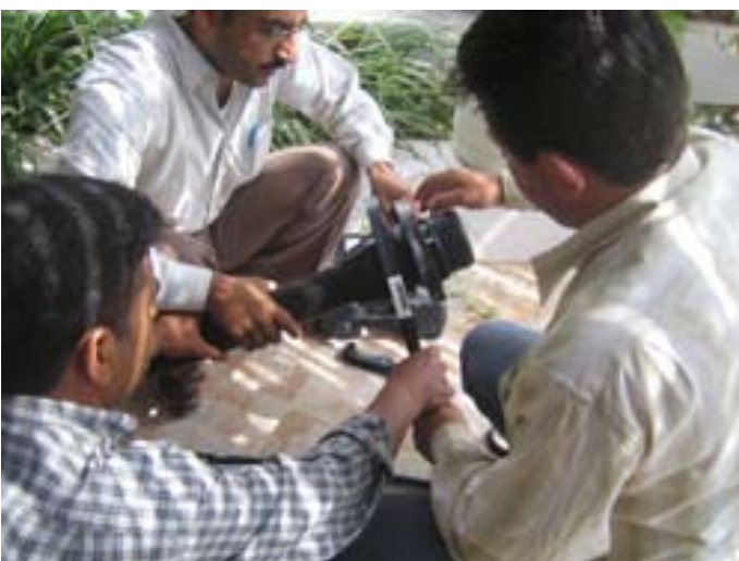
Practical installation of Fittingsinstall fittings
