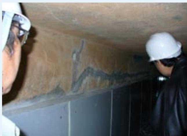
*Picture shows Mr. Nagasawa; Resident Representative inspecting Old Tunnel's Wet Periphery that has been coated with FRP Pannels, and one of the repaired cracks*
