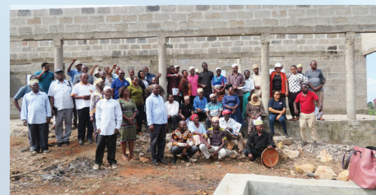
Dispensary which is being built by Community members.
