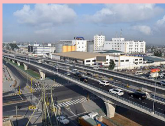
Mfugale Flyover in Dar es salaam
