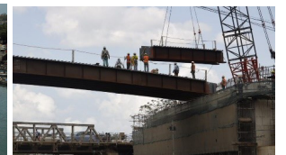
Mradi wa daraja la Gerezani, Dar es salaam
