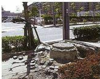
a manhole was lifted as a consequence of liquefaction
