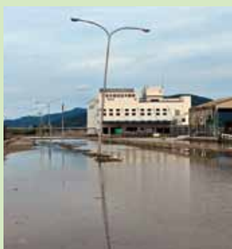
Port of Ishinomaki with ground subsidence
