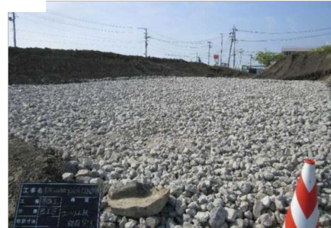
Debris is recycled for such as public work
