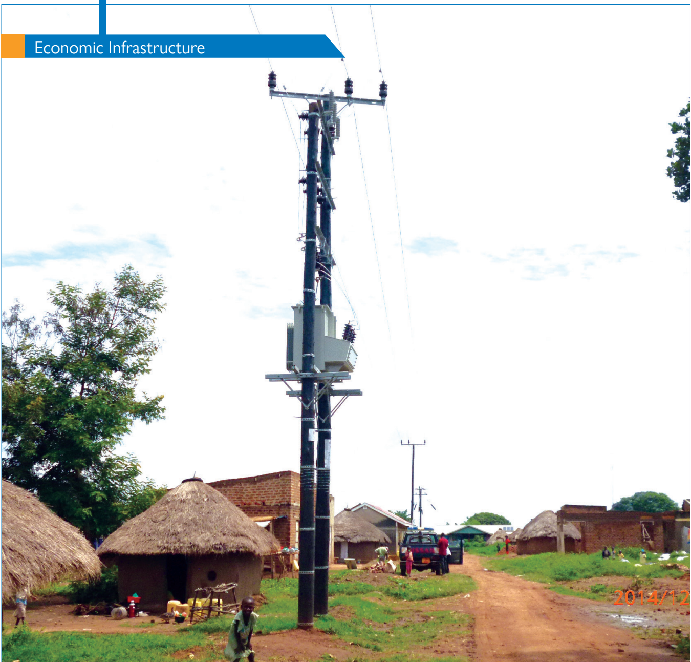
Low voltage line for the Rural Electrification Project Phase 3.
