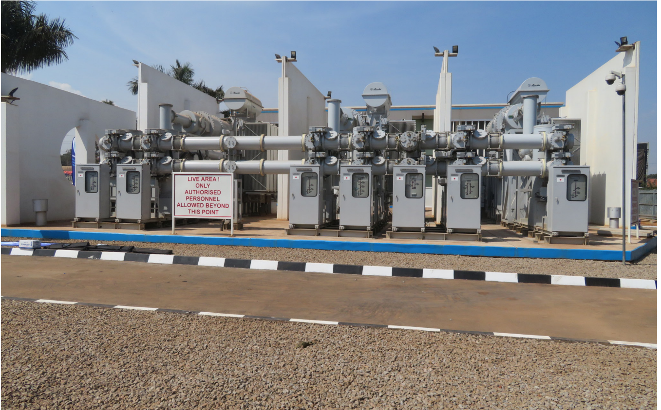
132/33kV Queensway Sub-station
