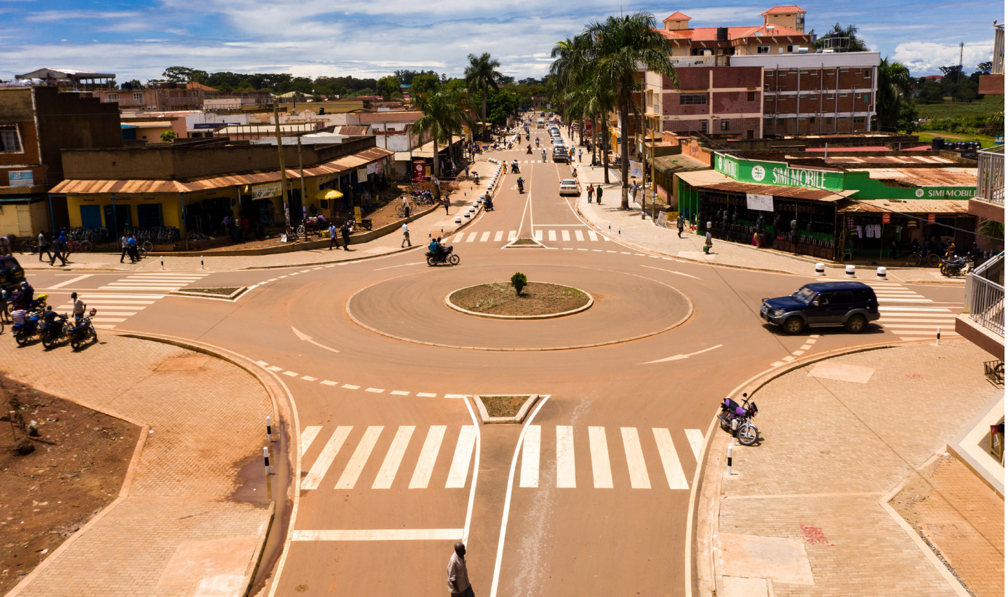
A roundabout built under the grant aid project for Improvement of Gulu Municipal Council Roads to ensure traffic safety.
