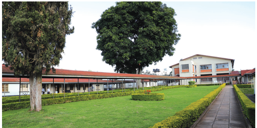
Kabale Referral hospital compound clean and well maintained
