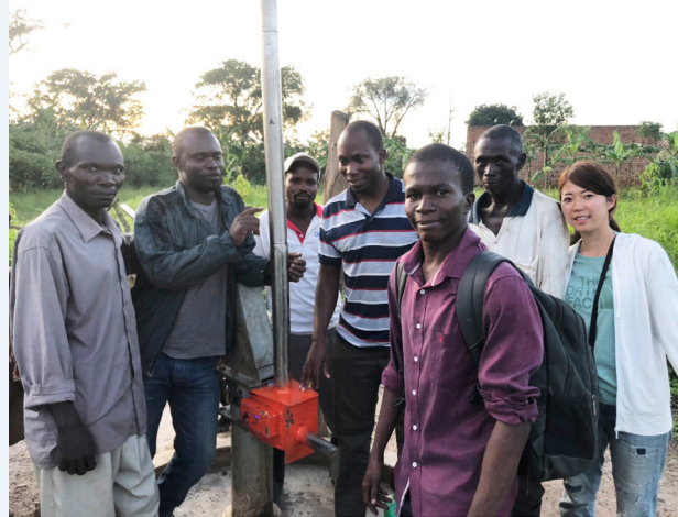
A JICA Volunteer with borehole technician and water user committee repairing a broken borehole in Gomba District.
