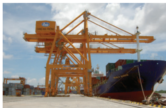
Rehabilitated Hai Phong Port
