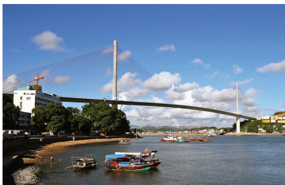
Bai Chay Bridge
