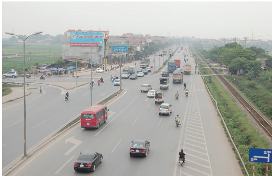
National Highway No.5 after improvement
