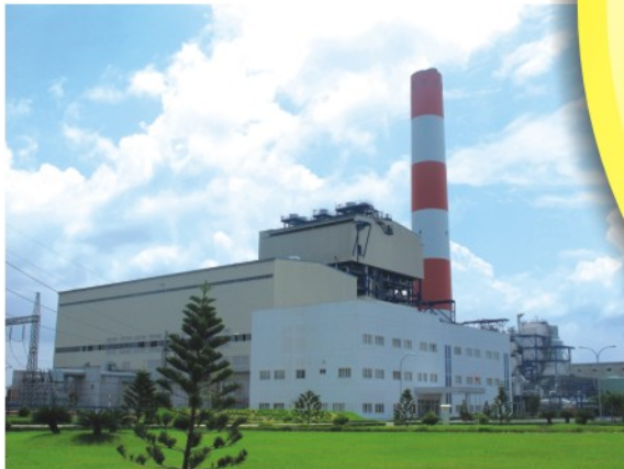
O Mon thermal power plant
