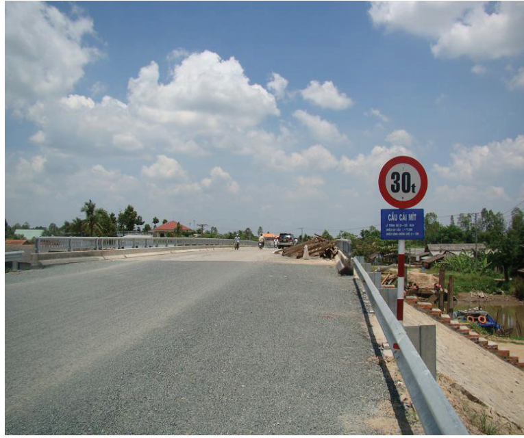
Cái Mít Bridge, Dong Thap Province
