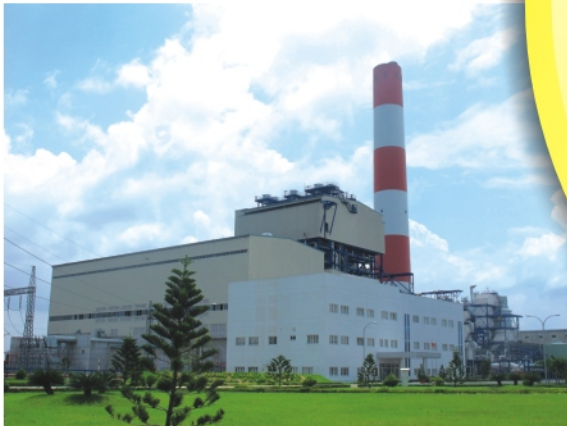
O Mon thermal power plant
