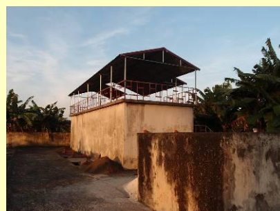
Water supply facility operated in proper manner as a result of the project
