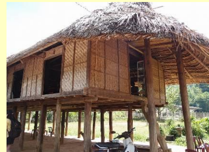
Community house constructed by villagers
