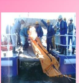
Installing an oil fence
