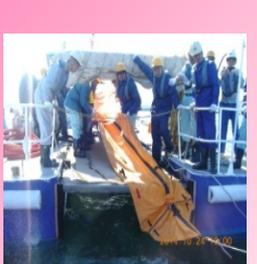
Installing an oil fence
