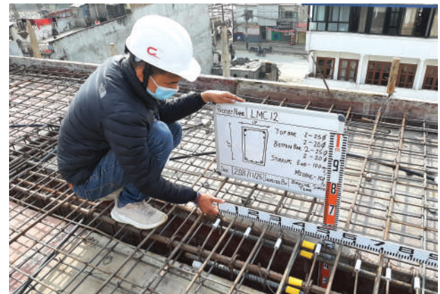
Checking reinforcement details of Beam
