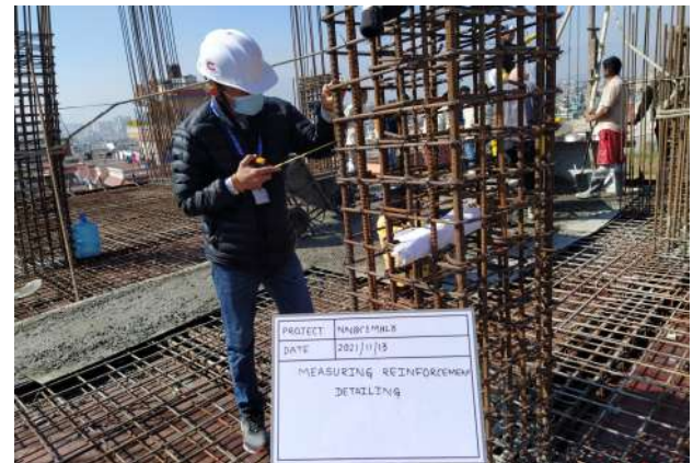
Checking reinforcement details of Column
