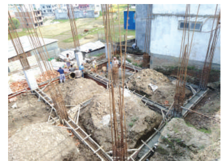
Ongoing construction sites
