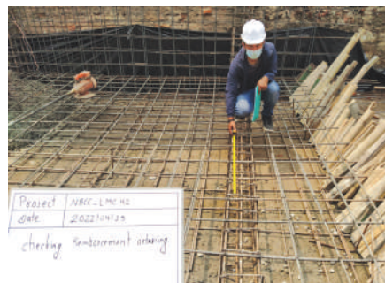
Checking reinforcement details of Foundation
