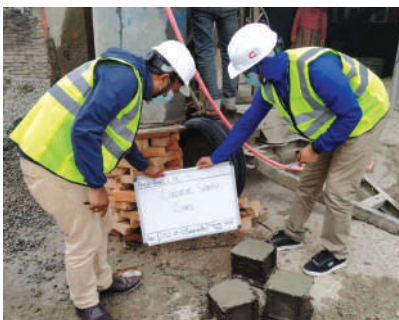
Collection of concrete test pieces
