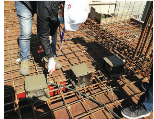
Collecting test pieces from the construction site
